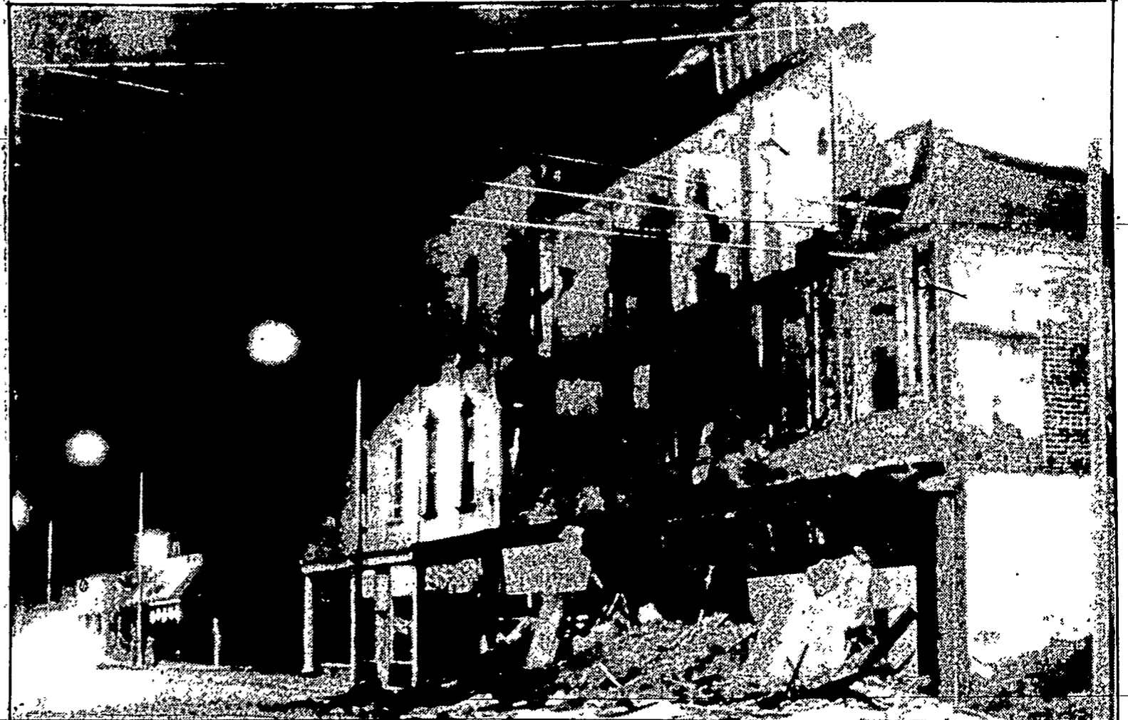
No injuries. At 10:30 last night the walls of the two upper levels of the Park House Hotel above the former Rod 'N' Gun tavern, in the 100 block of Washington Street, collapsed. Shown above is the damage which occurred.
